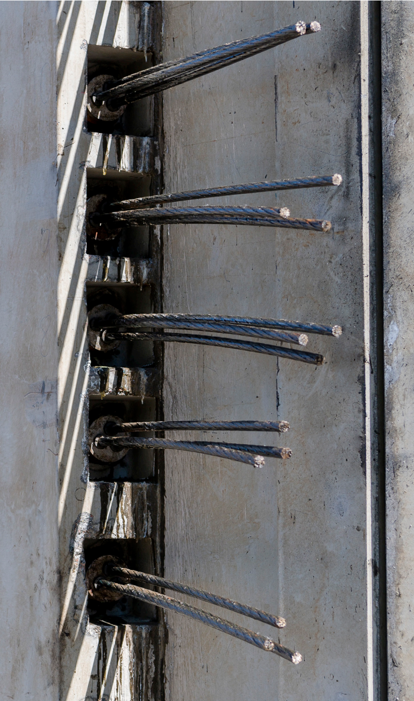
Tensioning elements on the C14 tank system.
